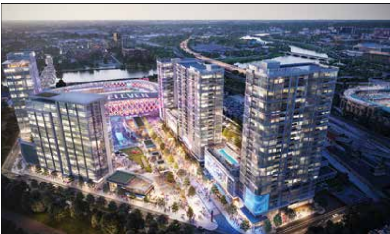
Eleven Park is anchored by a 20,000-seat multipurpose stadium that will be the new permanent home of Indy Eleven.
