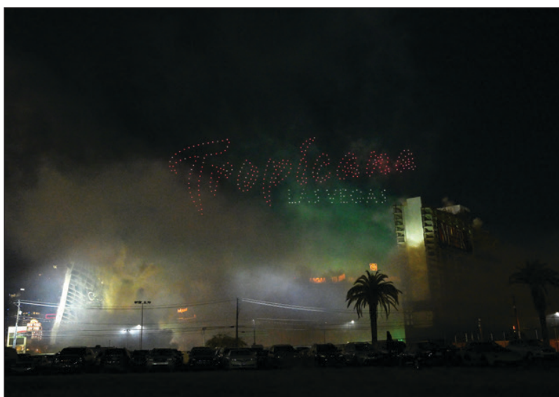
The Tropicana Las Vegas was demolished at 2:30 a.m. on October 9 following a fireworks and drone show. The implosion lasted 22 seconds, according to Bally’s Corporation, the property’s owner. The destruction of the long-standing Las Vegas Strip icon makes way for a forthcoming ballpark for the Oakland Athletics. Photo credit: Denise Truscello/Getty Images
