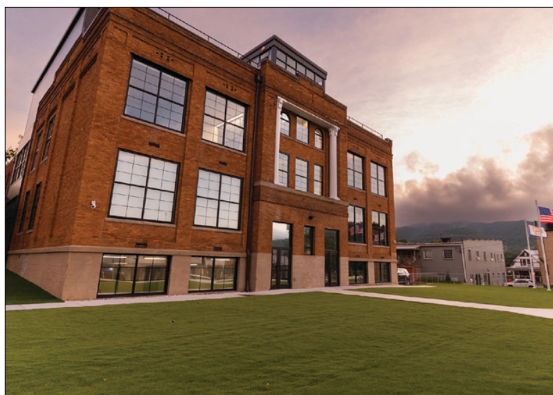
The Schoolhouse Hotel, Trademark Collection by Wyndham, a fully accessible hotel, launches the Accessibility Lab to test adaptive technologies.
