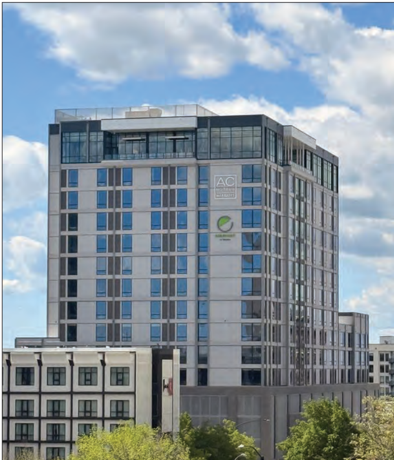
The dual-branded AC Hotels Boise Downtown and Element by Marriott Boise Downtown hotels are now hosting guests, developers announced on May 12.
