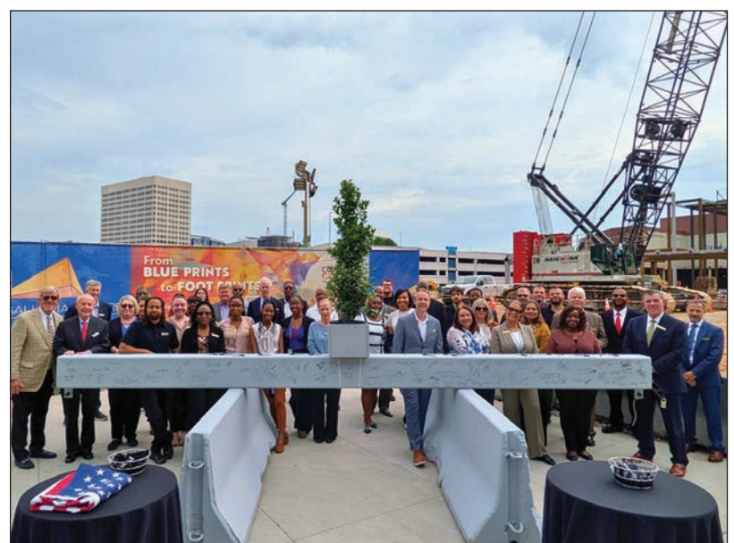
The Cobb Convention Center Atlanta in late May celebrated the placement of the final steel beam in its $190 million expansion and renovation project. The construction tradition of "Topping Out" saw members of the Cobb-Marietta Coliseum & Exhibit Hall Authority, the staff, and the construction team sign the final steel beam, which was also adorned by an American flag and a tree. The tradition of placing a tree atop a structure has its origins in Scandinavian culture, dating back over a thousand years.
