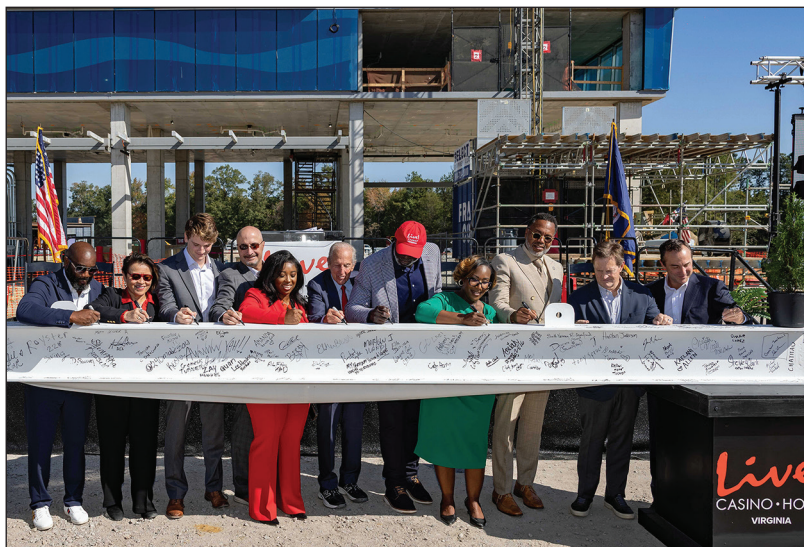
Representatives from the Cordish Companies and Bruce Smith Enterprise celebrated the topping out of the forthcoming Live! Casino & Hotel Virginia in Petersburg in early October. Officials gathered to sign the final construction beam before it was hoisted to its final position.
